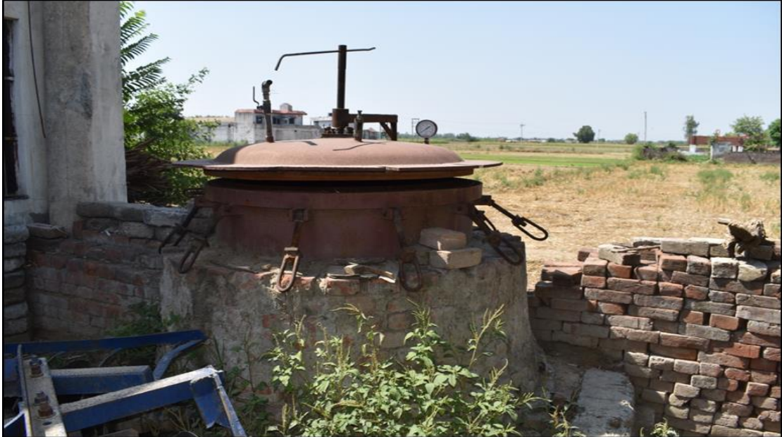
Figure 5.54: Traditional boiling vessel with pressure gauge at farmer's field in Punjab.
